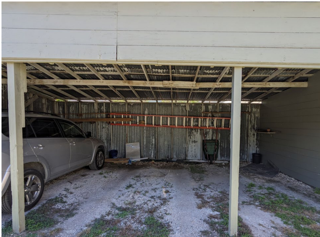
EAST (FRONT) ELEVATION – CLOSE UP
